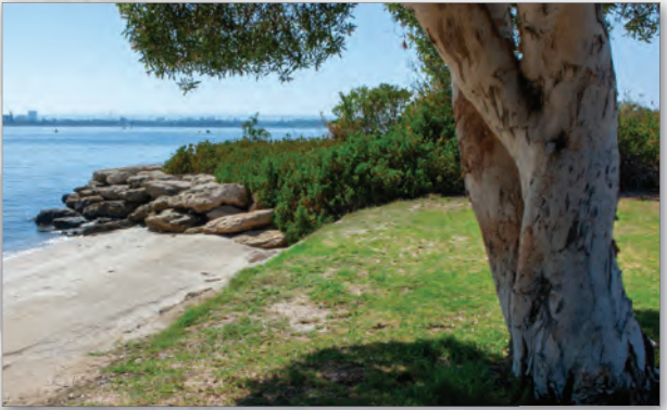
Planted groyne to replace existing sandbags
