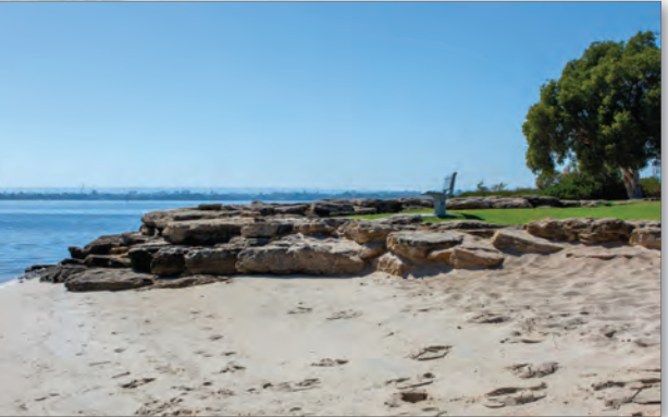
Groyne to replace existing sandbags
