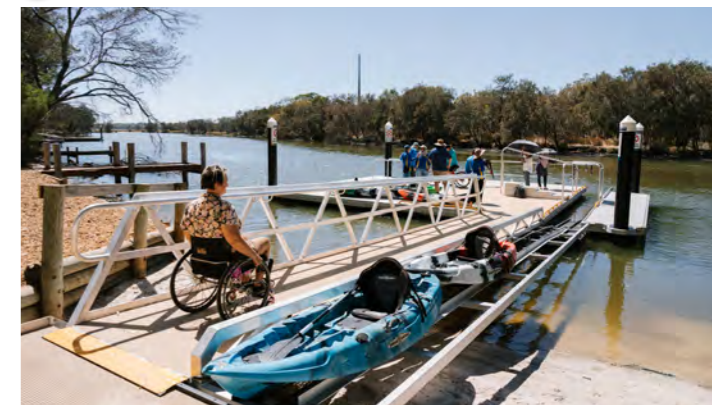
g All abilities paddle launch facility
