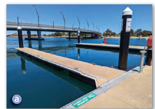
Commercial and Public Jetty
