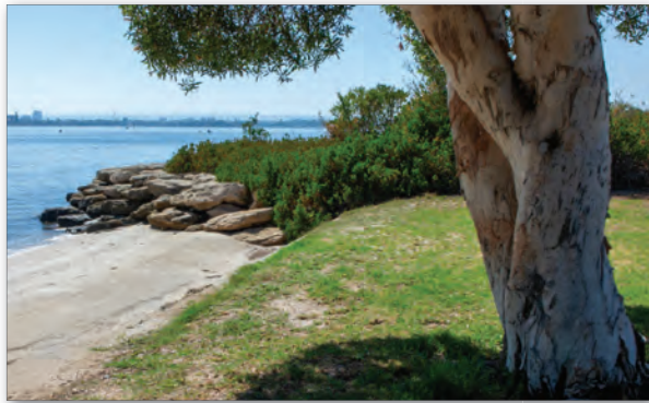
Planted limestone groyne to replace existing sandbags on Western Foreshore
